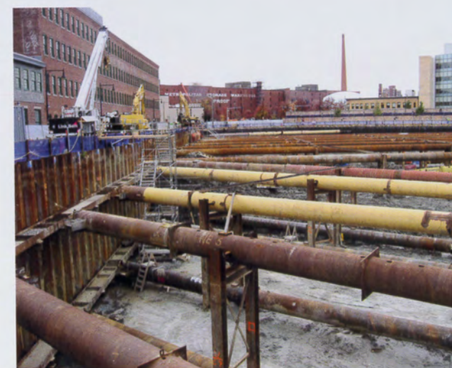
Deep foundation support at Novartis Campus, Cambridge, MA
